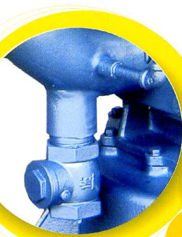
逆轉保護裝置 Reverse Rotation Protection Device
